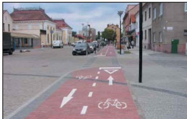
An example of cycle track constructing in Hodonín
